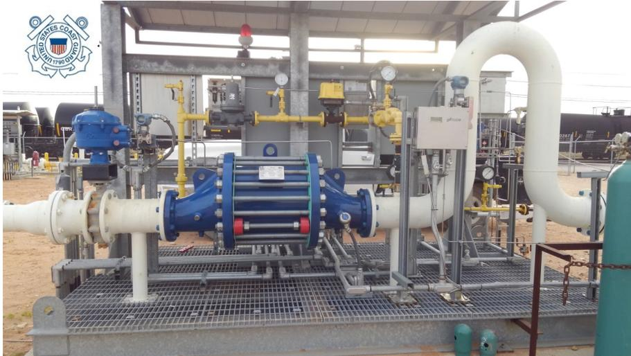
*The Paradox Detonation Flame Arrestor* represents the best technology for value in flame arrestor protection. They prevent flame propagation by absorbing heat and dissipating supersonic pressure waves, using multiple spiral wound crimped ribbon flame cells staged with turbulent creating
